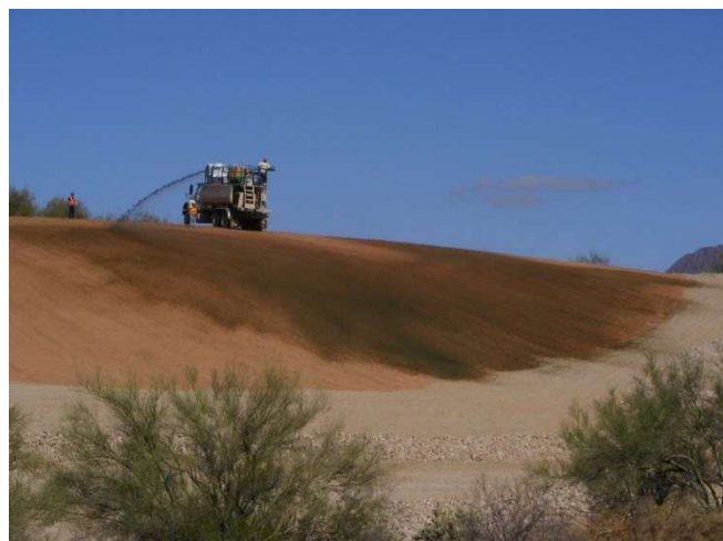
Figure 1.4: Revegetation efforts on top of repository cap [2].
