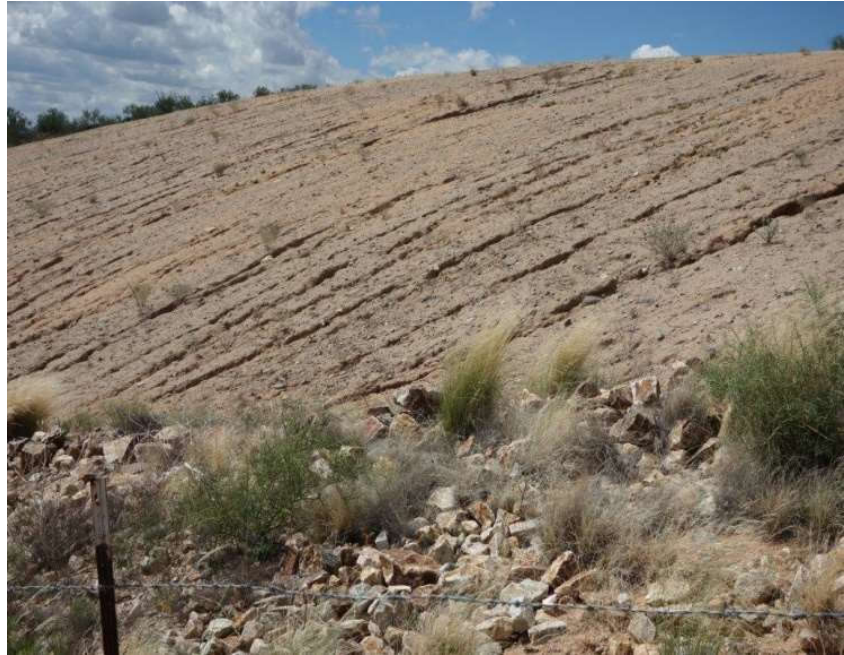
Figure 1.5: Vegetation is sparse and erosion is evident on the repository cap [6].
